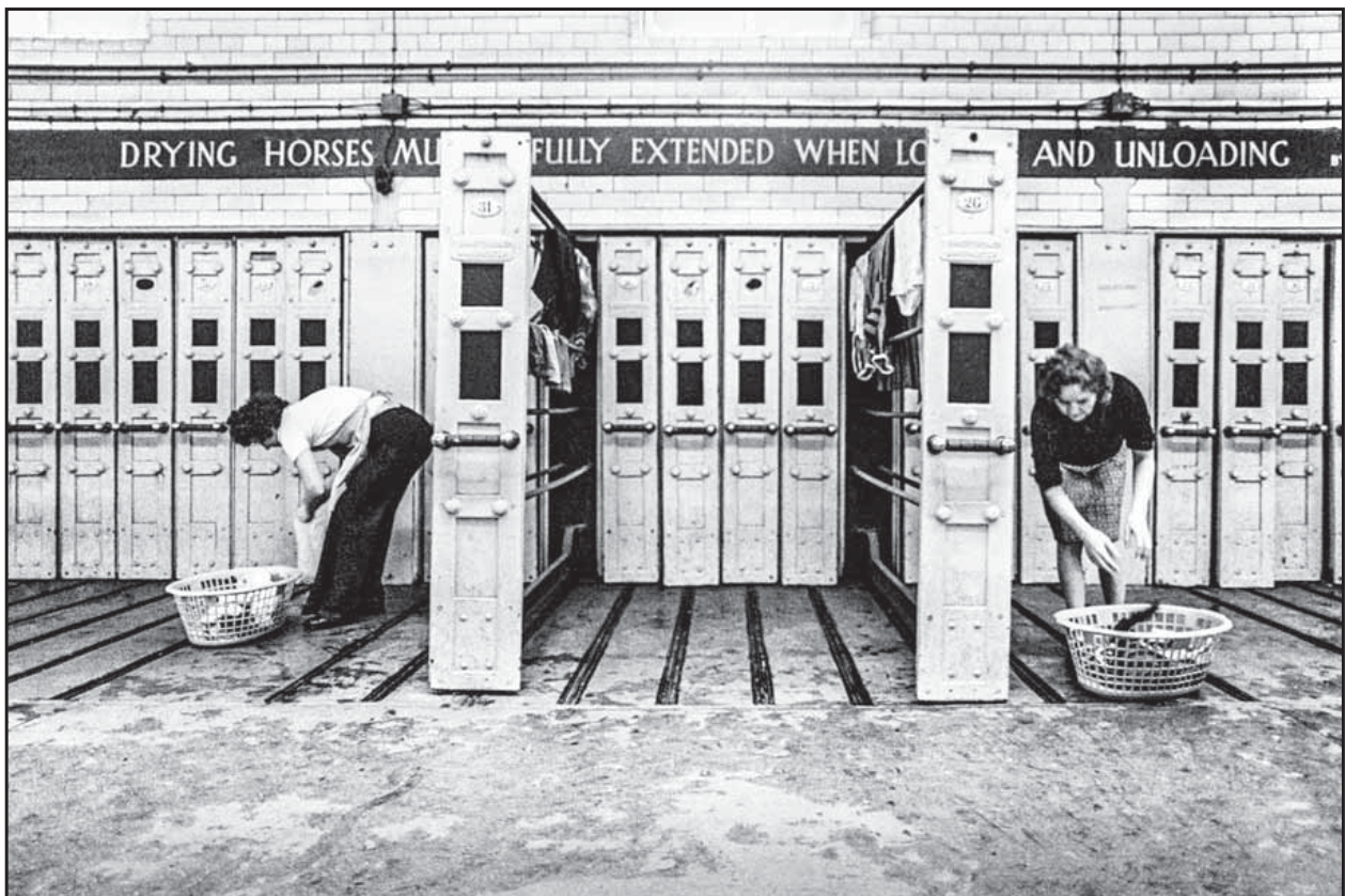
Fig. 8. Interior of McLeod St Public Washhouse. Photograph showing drying horses, 31 March 1977. (Courtesy Brian Scotchburn Snell, photographer.)
